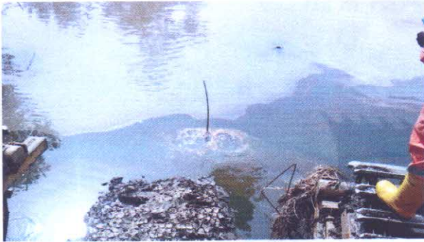
SPILL POINT BEFORE EXCAVATION
