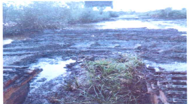
BACK FILLING OF SPILL POINT
