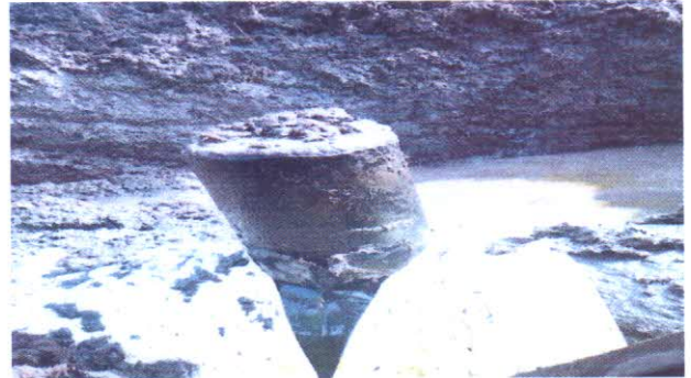
SPILL POINT AFTER EXCAVATION
